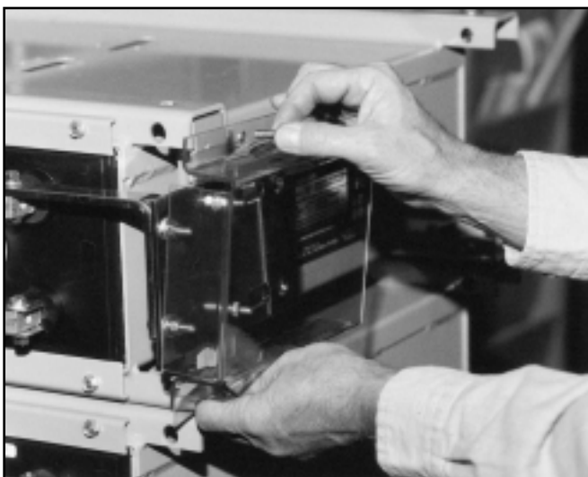
Fig. 18 (Side Terminal Plate Shield Assembly)
