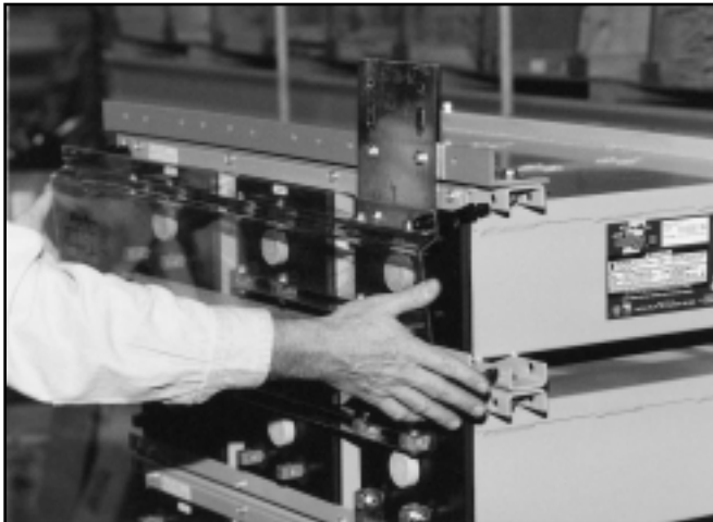
Fig. 17 (Front Shield Assembly)
