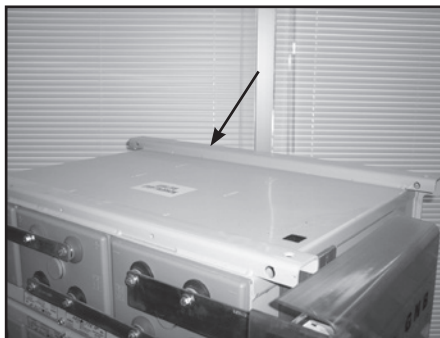
Figure 4: Recommended Frame Ground Location
