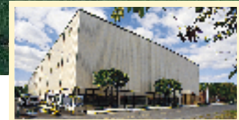
Cable and Wire Plant
